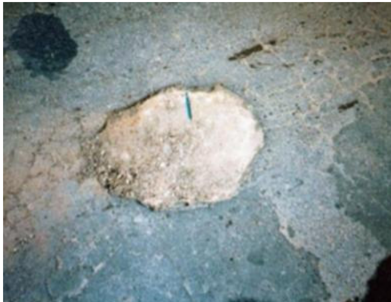
Figura 17: Panela (P)
