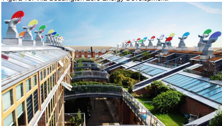
Figura 15: Vila Beddington Zero Energy Development .
