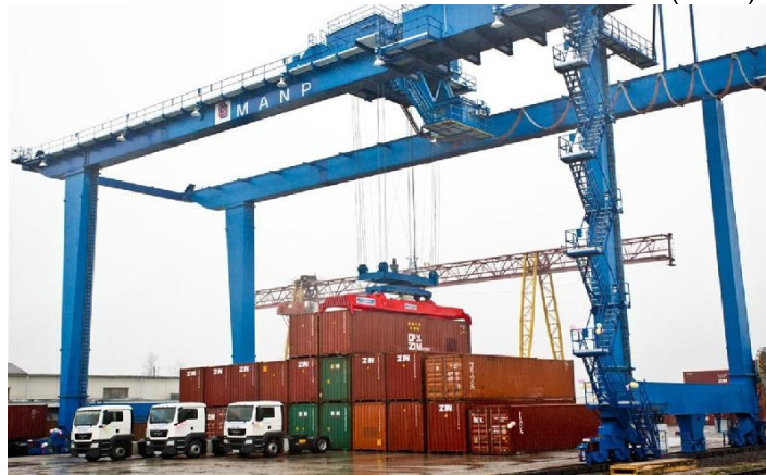
FIGURA 5 - RAIL MOUNTED GANTRY CRANES (RMG)
