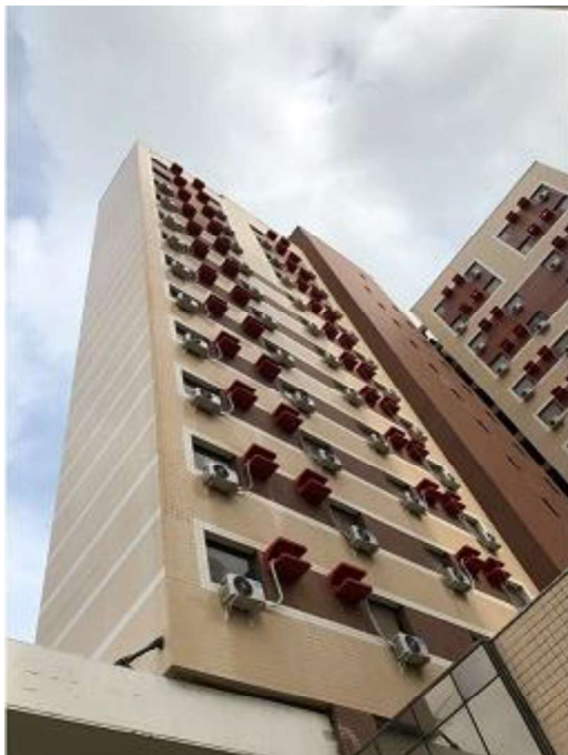
Figura 1- Fachada do Hotel Soft Win
