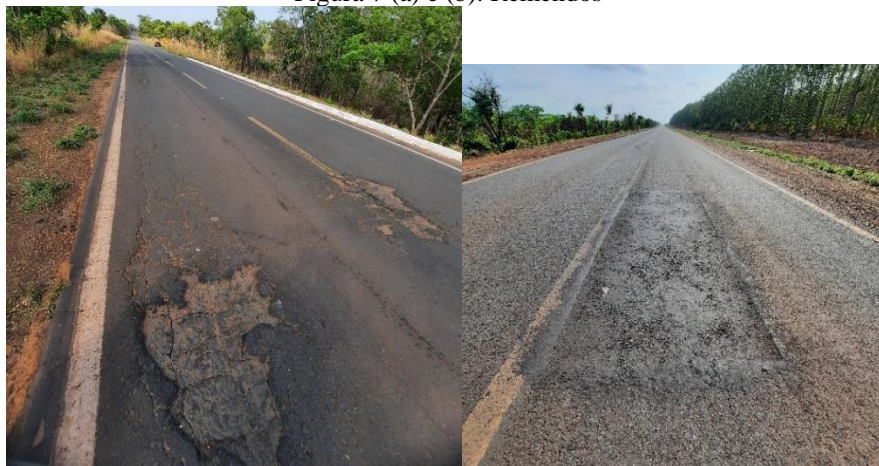
Figura 7 (a) e (b). Remendos
