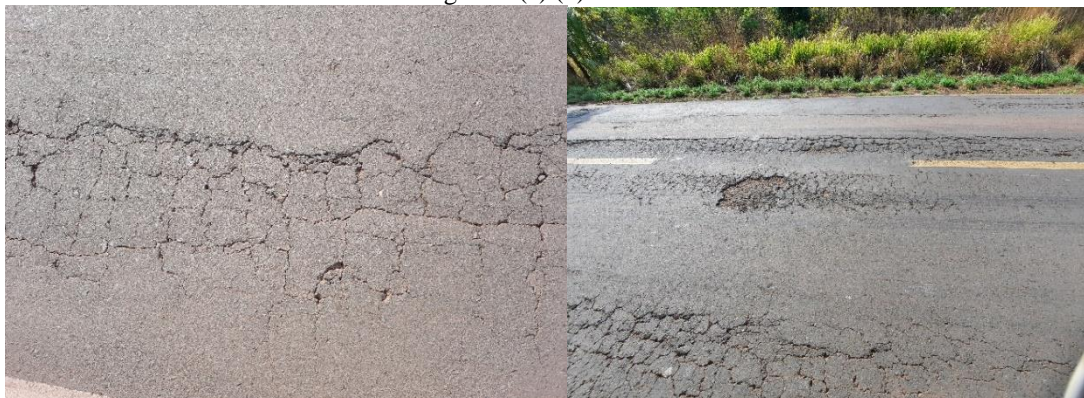
Figura 9 (a) (b). Trincas
